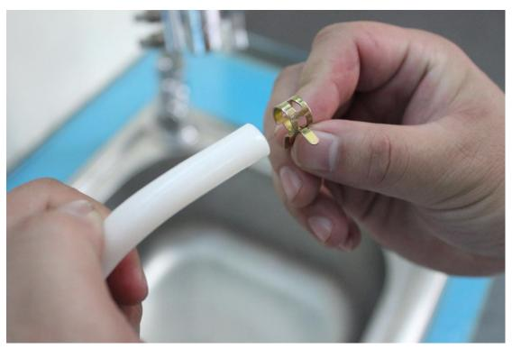
Fix the metal pipe clip to the other end of water pipe which is from the pre-filters outlet.
