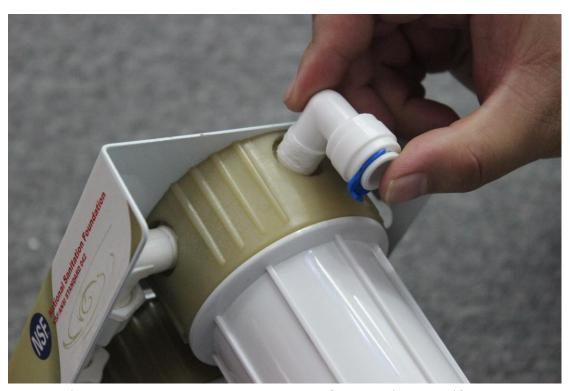
Connect the easy connector. Use some water proof tape on the screw if necessary.
