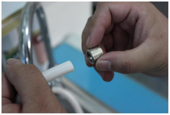
Put the end of water pipe(which is connecting to the water inlet on the pre-filters.) through the screw nut.
